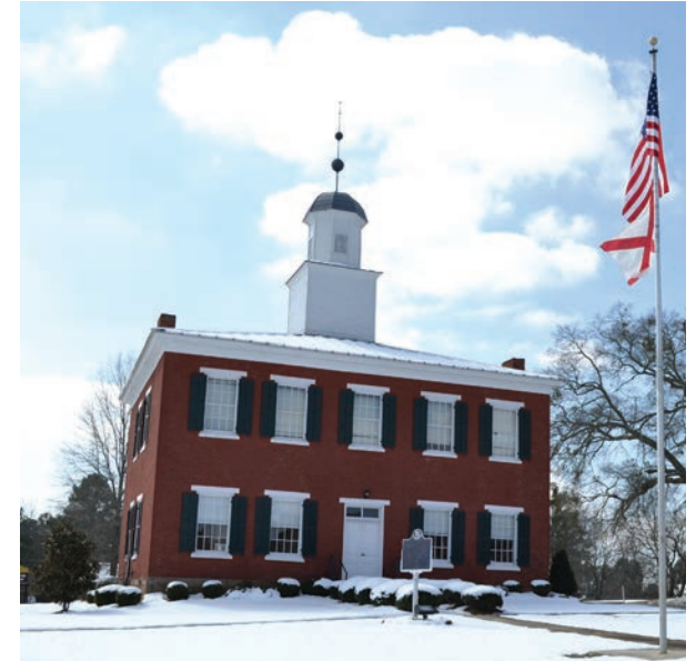
Old Morgan County Courthouse in Somerville
