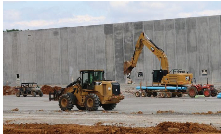
First Solar plant under construction
