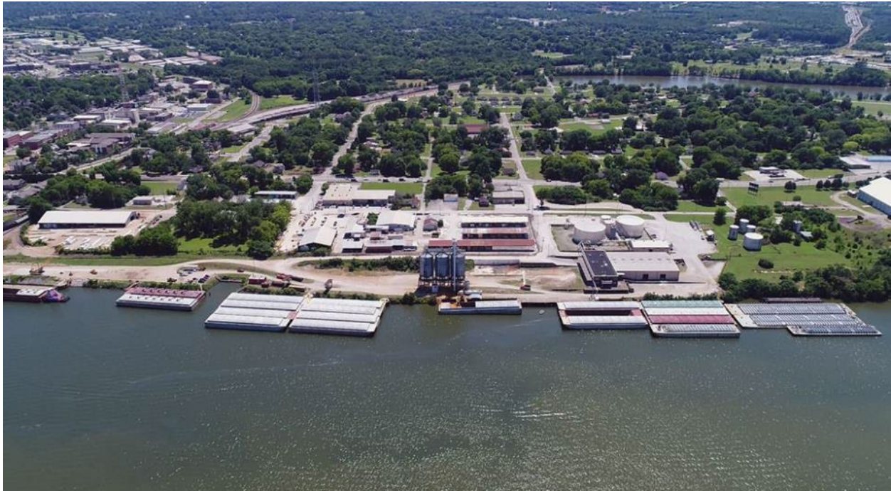
Source: Aerial Photo of Decatur Morgan County Port Authority Alabama
