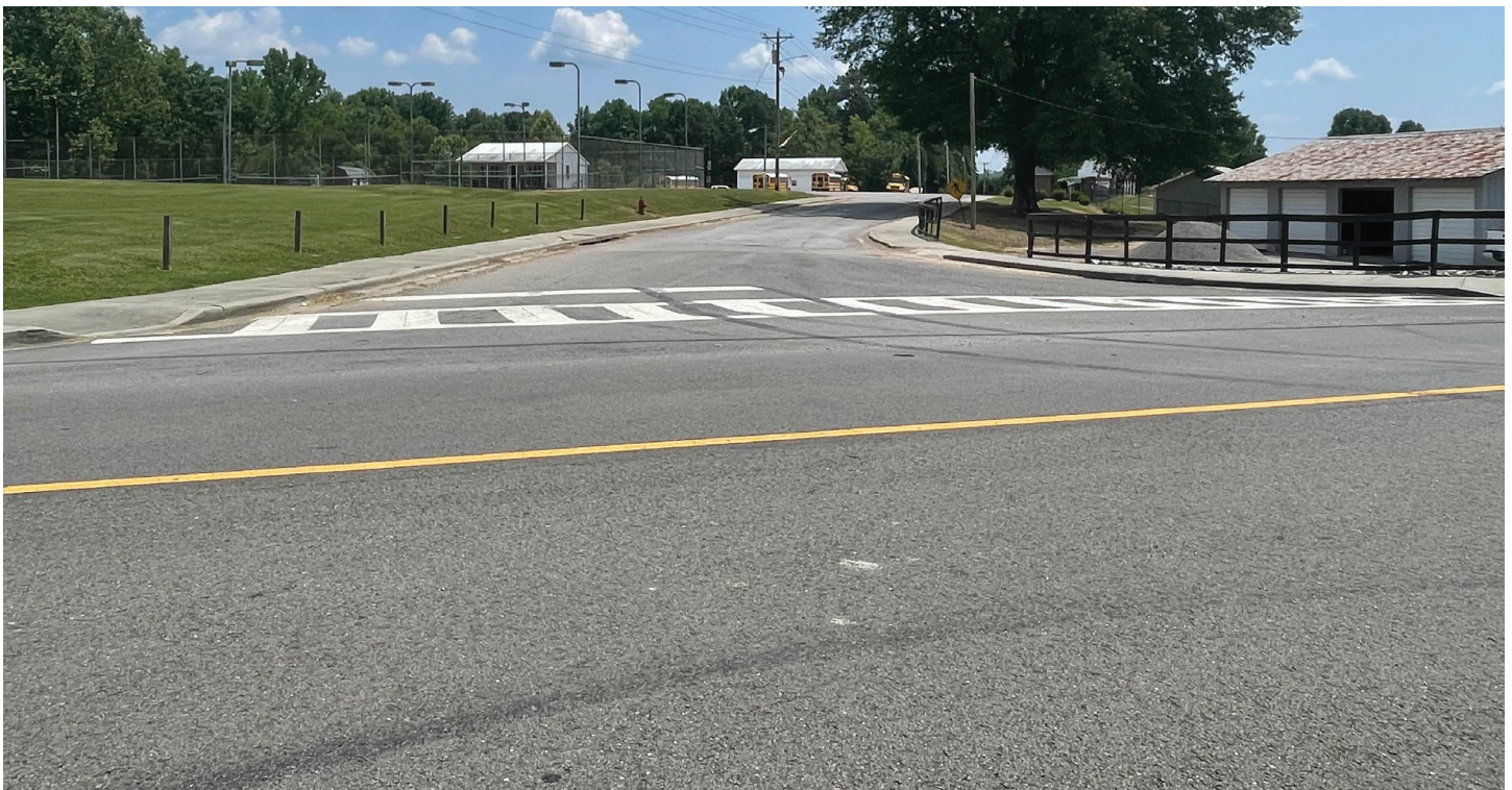
Looking south at intersection with County Road 1140
